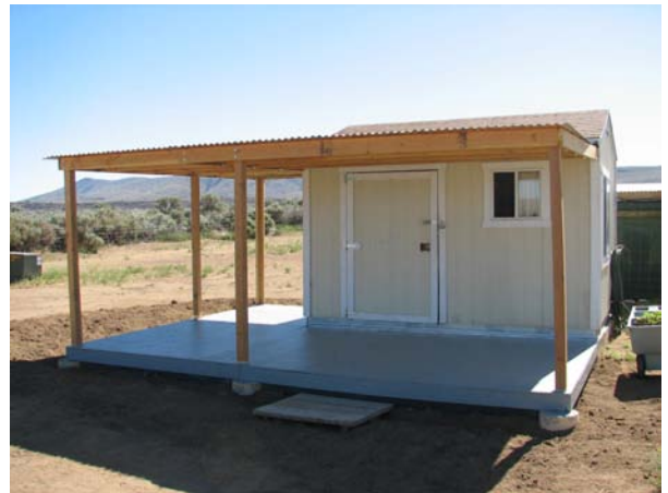
Completed ! Keeps us more comfortable in the summer!
