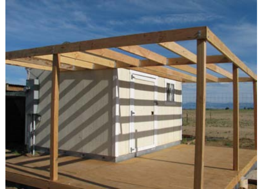
Bunkhouse porch, phase 2
