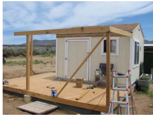
Bunkhouse porch, phase 1
