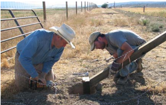
Bracing placement for the gate with our nephew Asaf.
