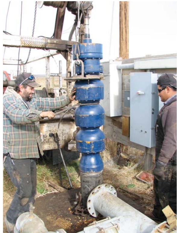
The new pump is carefully guided & secured into place.
